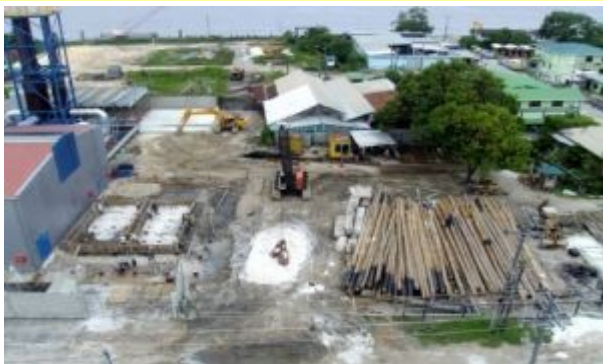
Foundation work in progress for the new GPL generators - GPL pix
